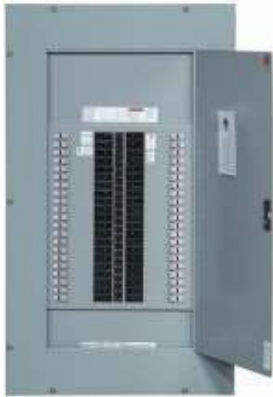
Type PRL1a Panelboard
